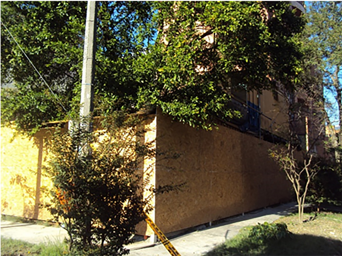
Figure 10. New temporary site enclosure.
