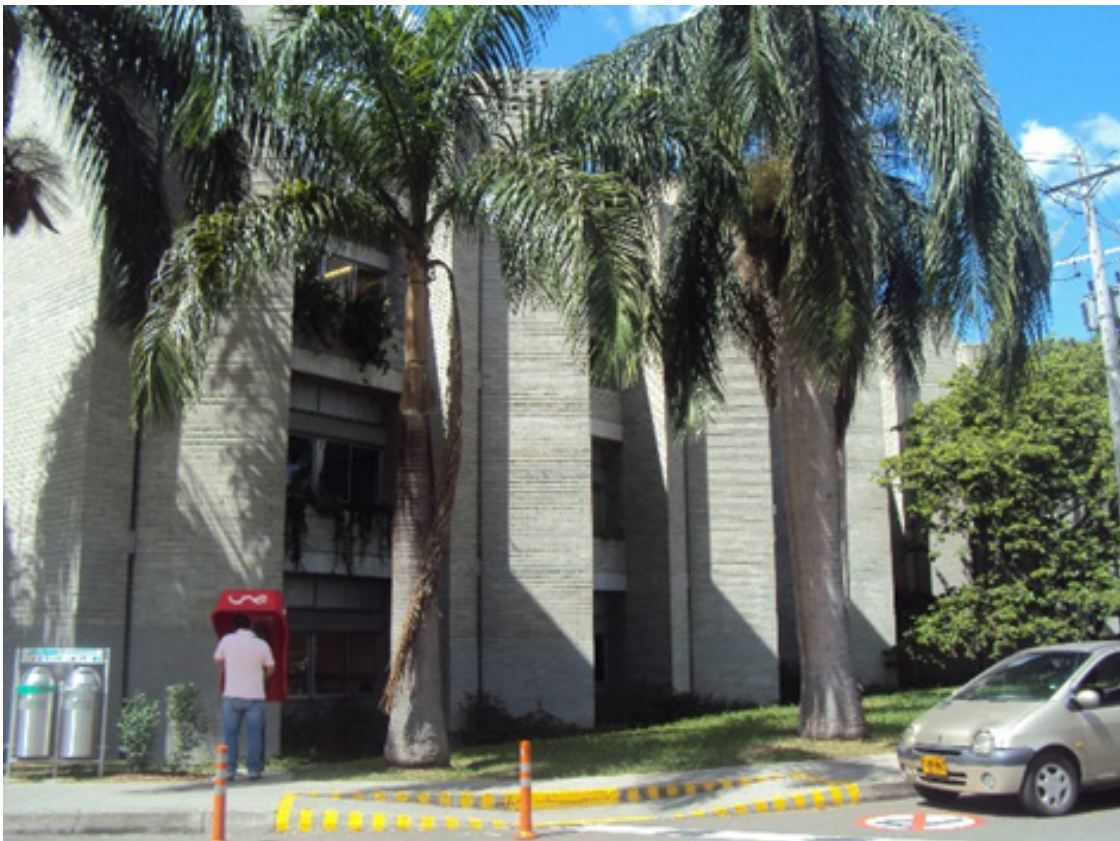
Figure 2. Block 19a in the Universidad Nacional de Colombia Campus Medellín; recycled concrete block walls
