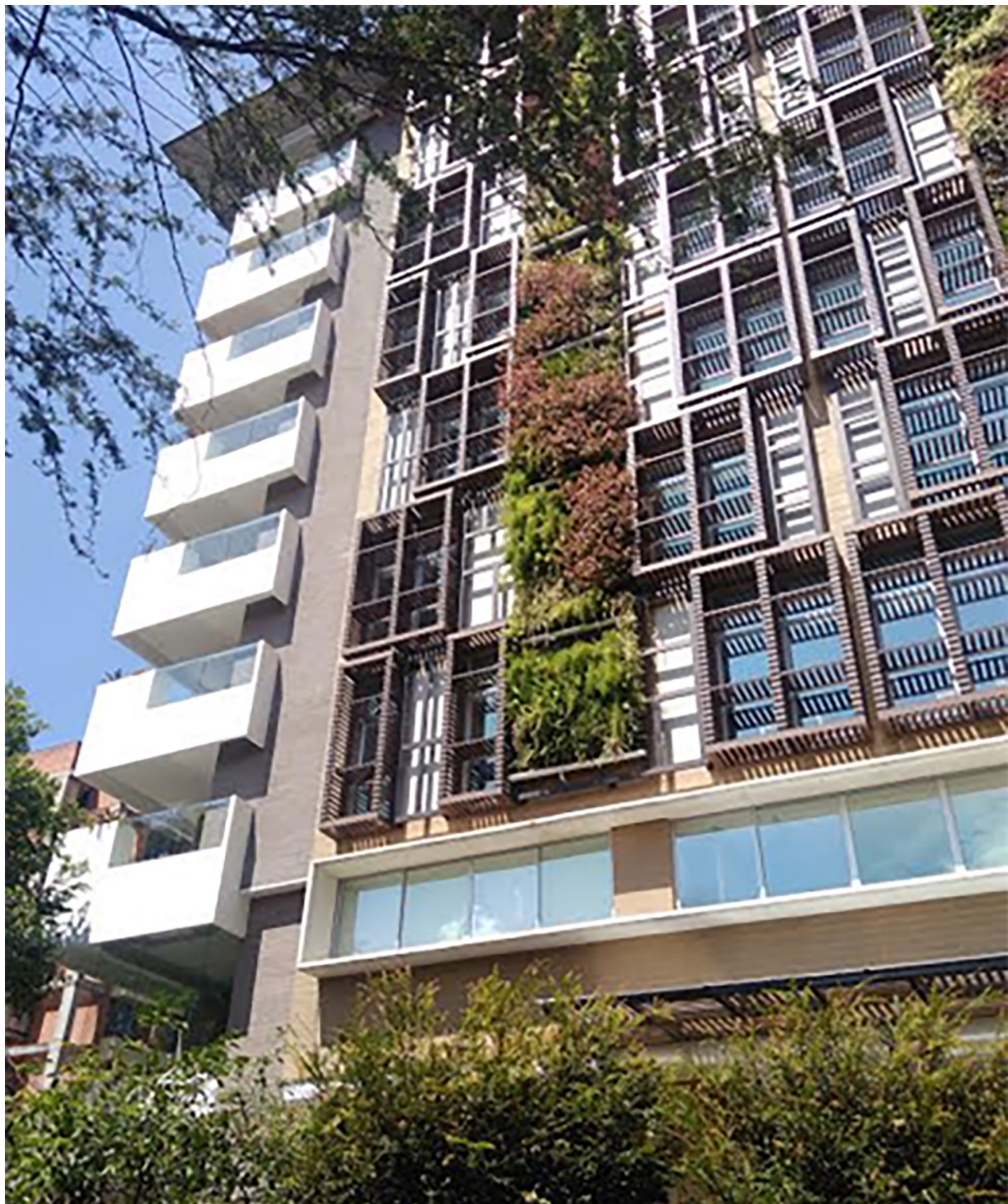
Figure 12. Façade with sunbreaks and landscaped walls.
