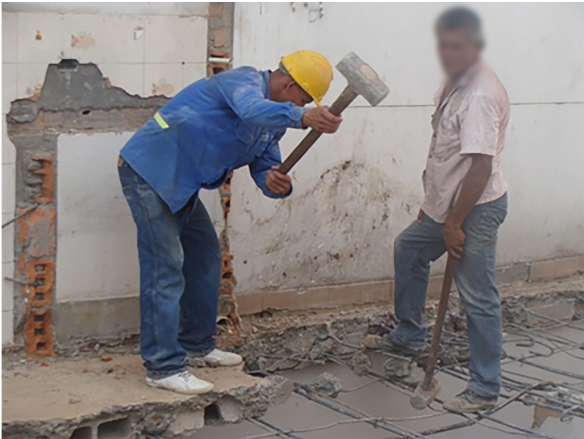
Figure 9. Workers without occupational health and safety conditions.
