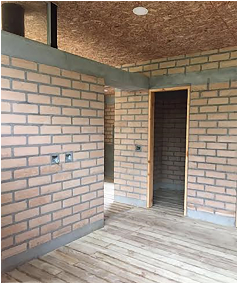
Figure 20. SCB and reinforced concrete beams.
