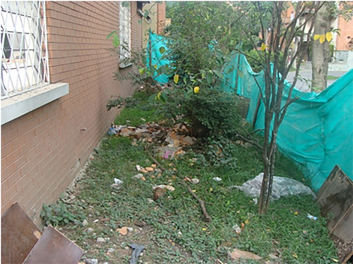
Figure 7. Unsafe and unsightly enclosure.
