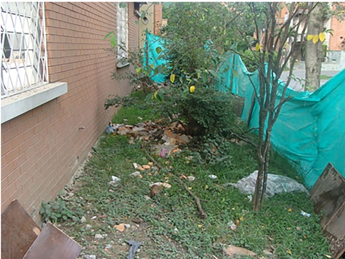
Figure 7. Unsafe and unsightly enclosure.
