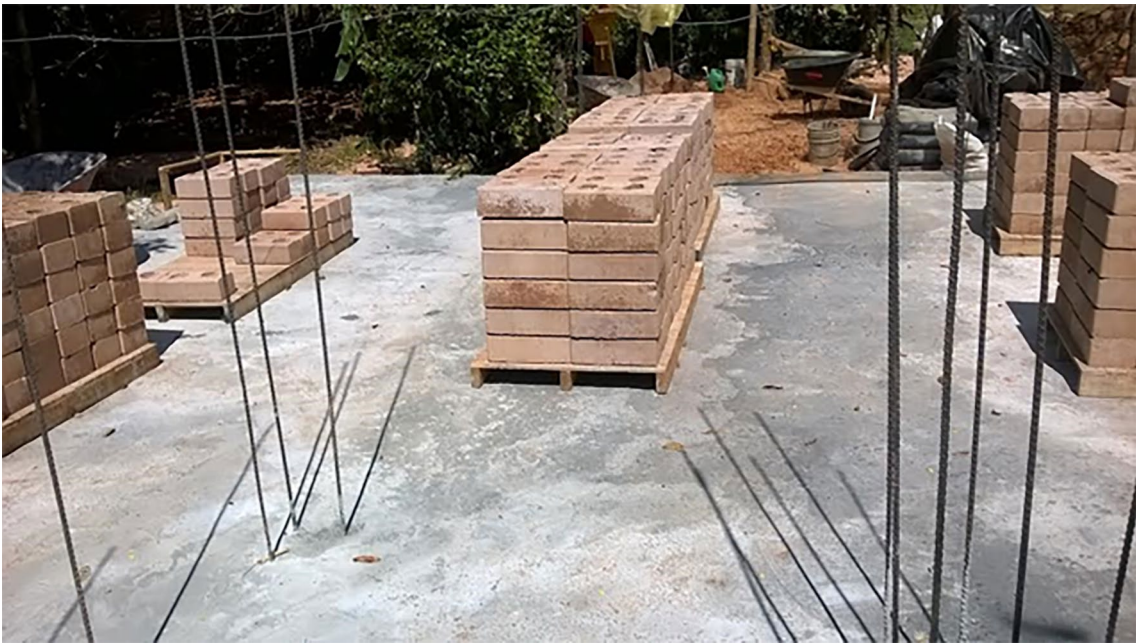
Figure 19. SCB made on site.
