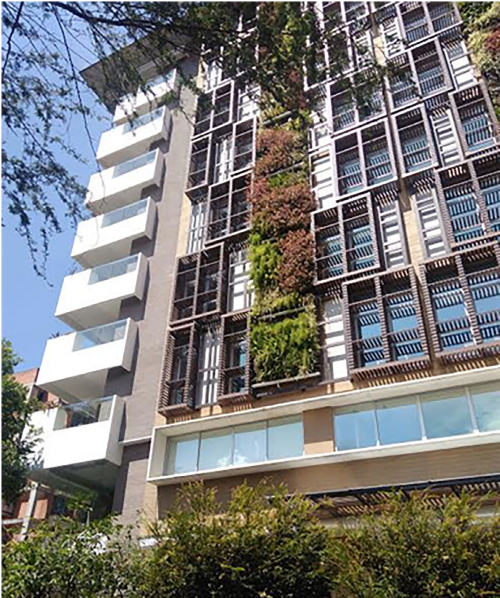
Figure 12. Façade with sunbreaks and landscaped walls.
