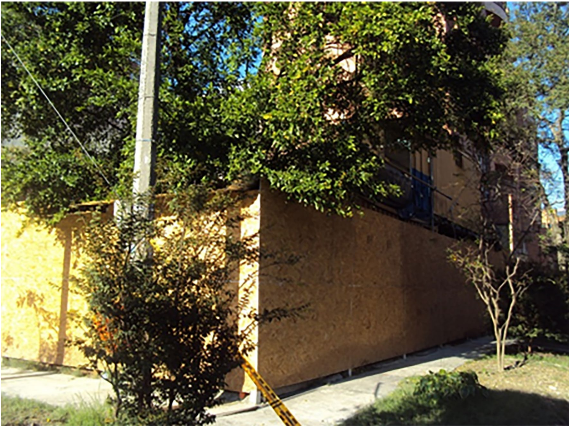
Figure 10. New temporary site enclosure.
