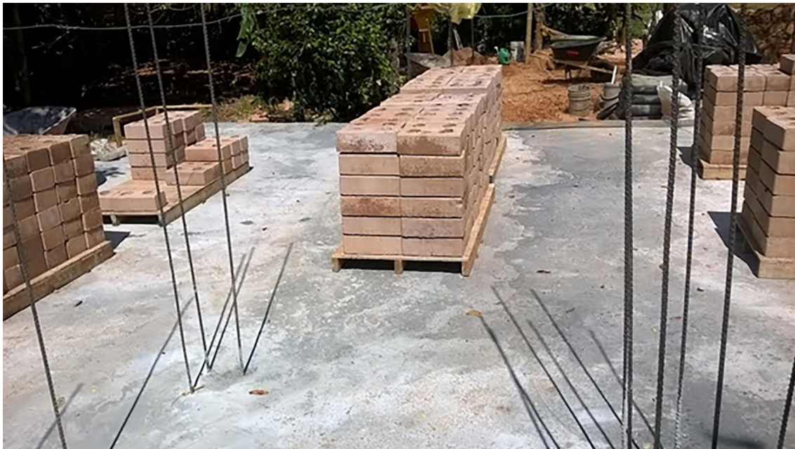
Figure 19. SCB made on site.
