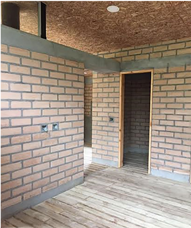
Figure 20. SCB and reinforced concrete beams.
