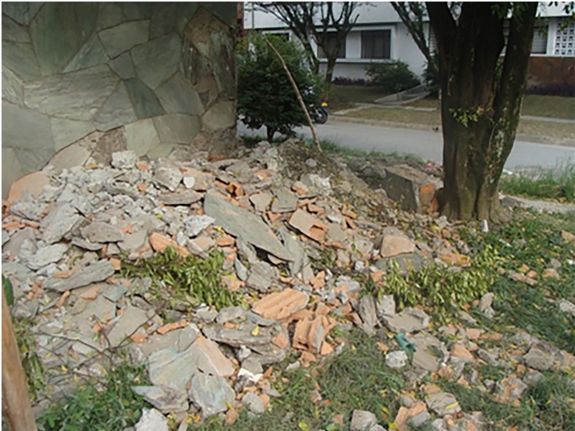
Figure 8. Inadequate disposal of CDW at the construction site.
