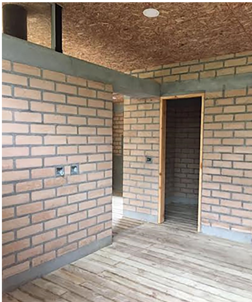
Figure 20. SCB and reinforced concrete beams.
