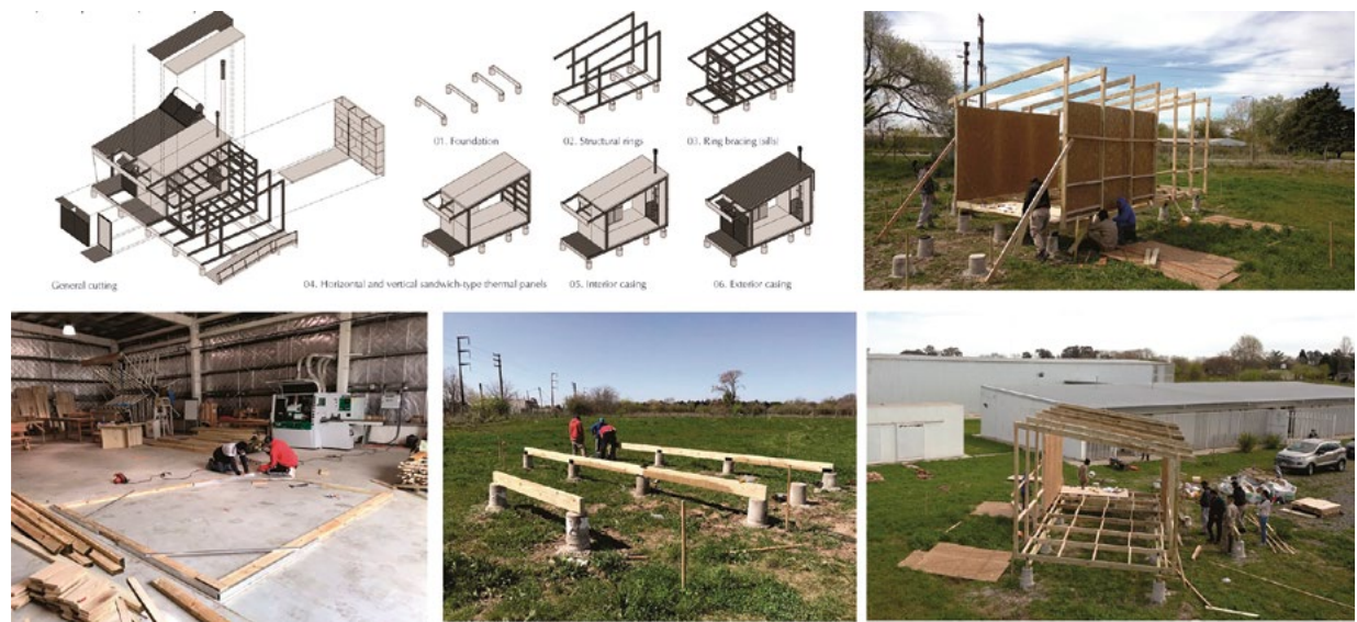
➤ Figure 7. Resistant spatial structure; quartering; progressive assembly, and participative management of the local work cooperative, the technicians of the IIPAC-FAU-CONICET-UNLP and the Centro de Tecnología en Madera (CTM) of the UNLP. Source: own elaboration (2021).
