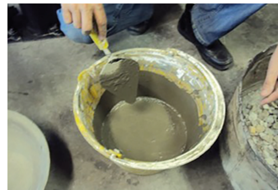
Figure 8. Mixing cement with water: mechanical suspension. Source: own elaboration (2019). CC BY
