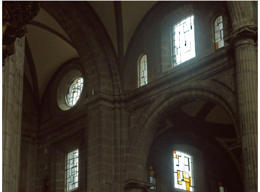
Figure 8. Interior of the Metropolitan Cathedral of Mexico City, showing the current view of the stained glass windows designed by Mathias Goeritz Source: Cedeño, 2015.
