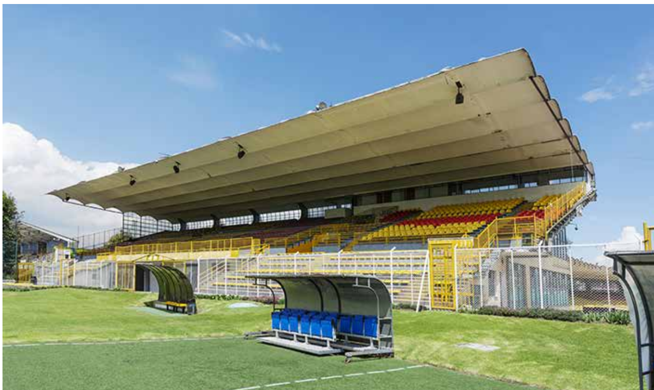
Figure 14. Current view of the main grandstand of the Hippodrome of Techo Source: Own elaboration, 2018, CC BY.
